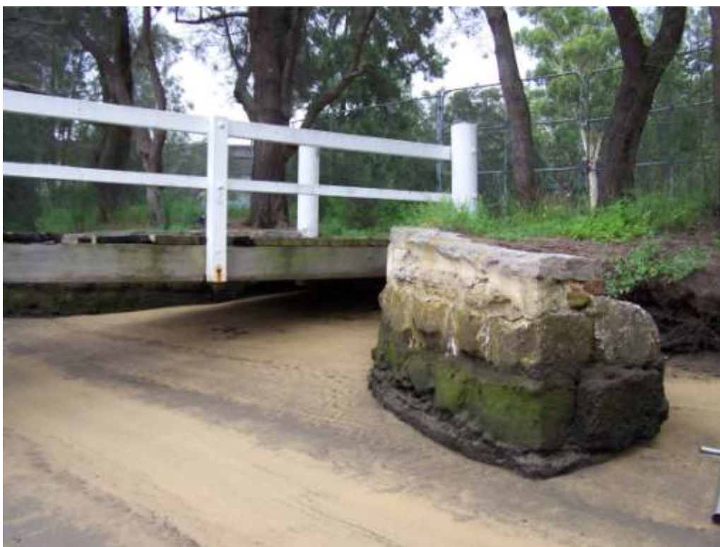
Image: Cairds Wharf *Remains of the original wharf in this picture are not located in their original location. The wharf in this image was built in 1981.
