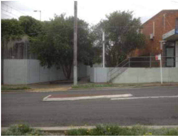
Image: Entrance to East Hills Station from Maclaurin Avenue
